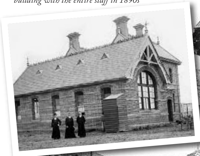
Below: The original Assumption College building with the entire staff in 1890s
